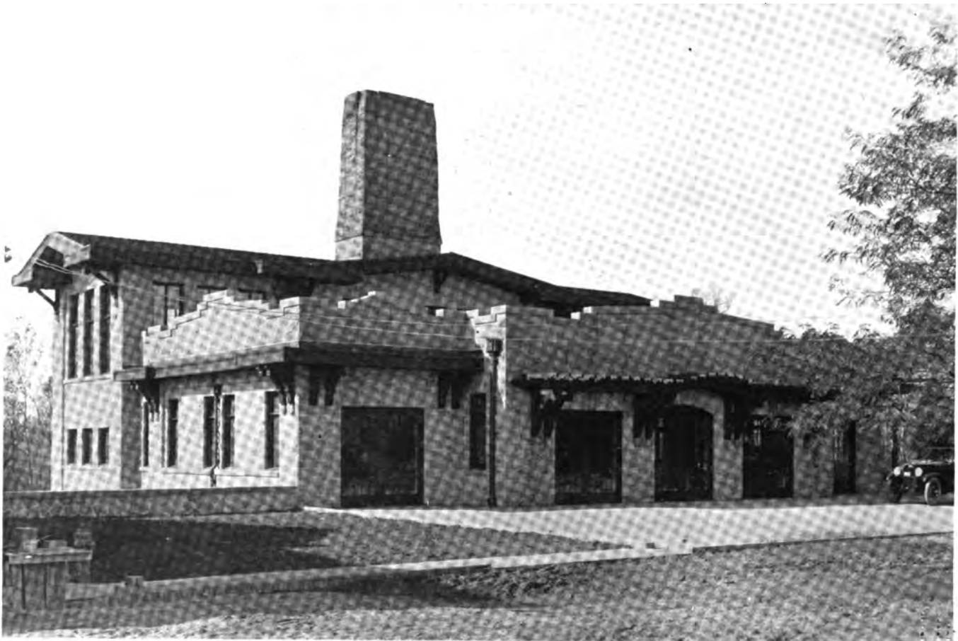
Garage, Power House and Laboratory. HOUSE, HENRY FORD, DEARBORN, MICH.
